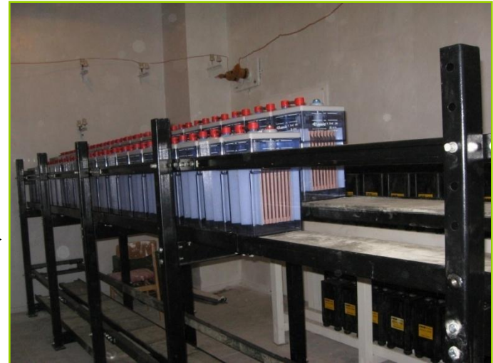
New storage battery of new system of emergency power supply (SEPS)
