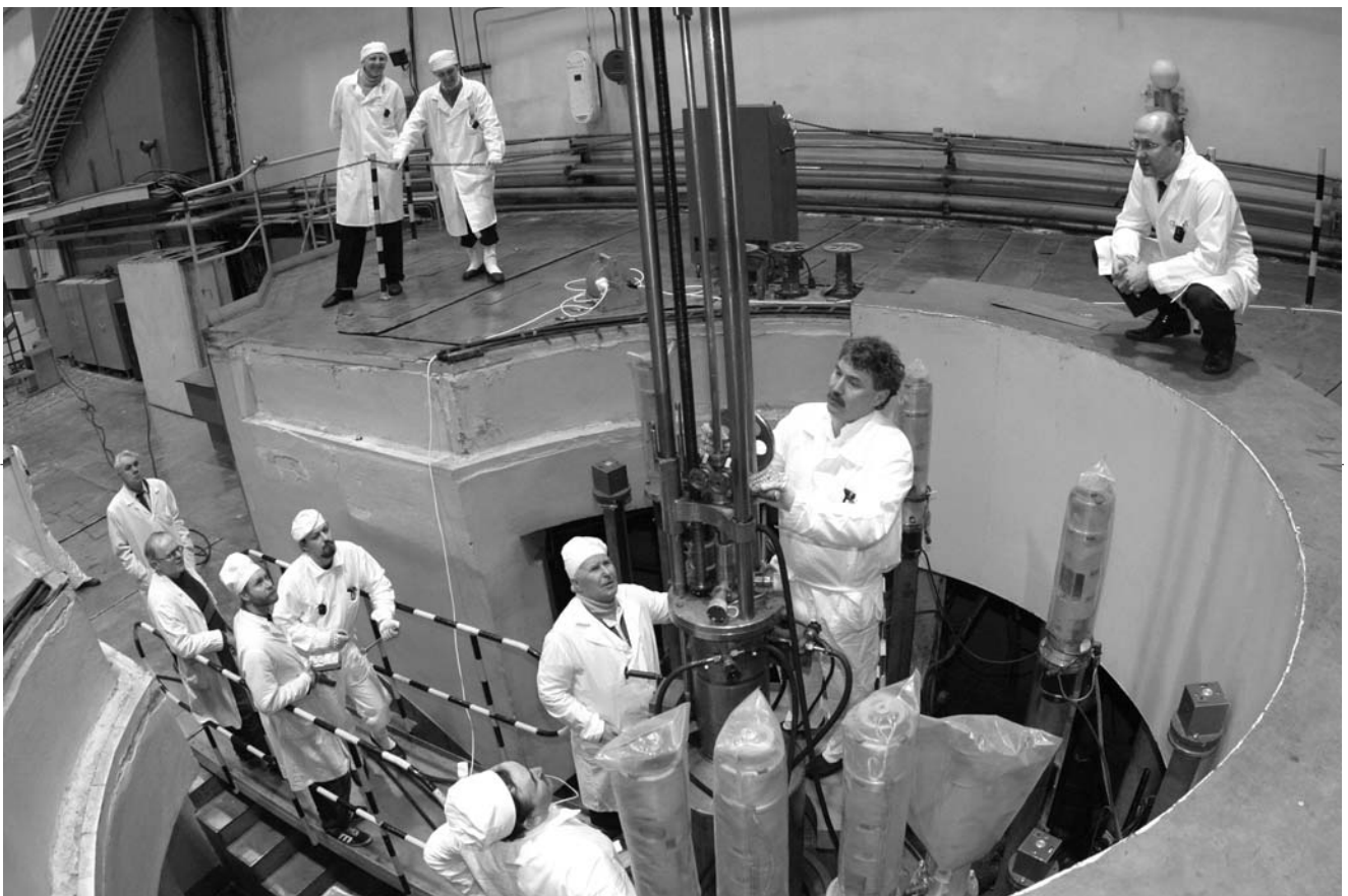
Frank Laboratory of Neutron Physics, March. Unloading the IBR-2 reactor active zone
