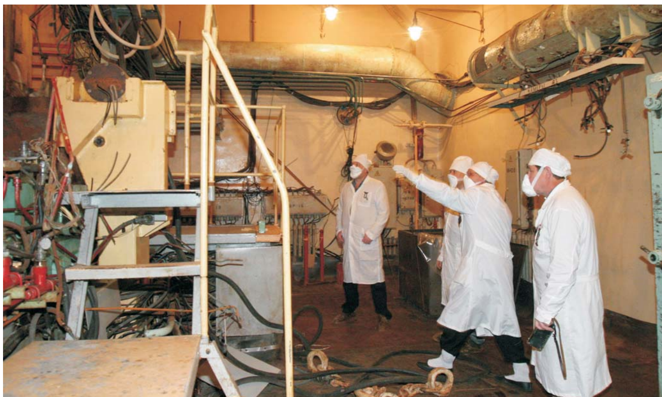
Frank Laboratory of Neutron Physics, October. IBR-30 dismantling
