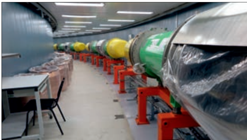
Magnetic cryostat system of the NICA Booster is being assembled
