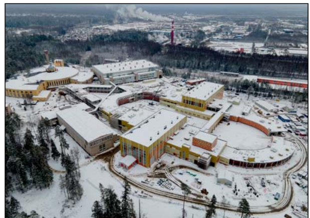
Fig. 3. General view of the construction site of the collider complex (November 2020)
