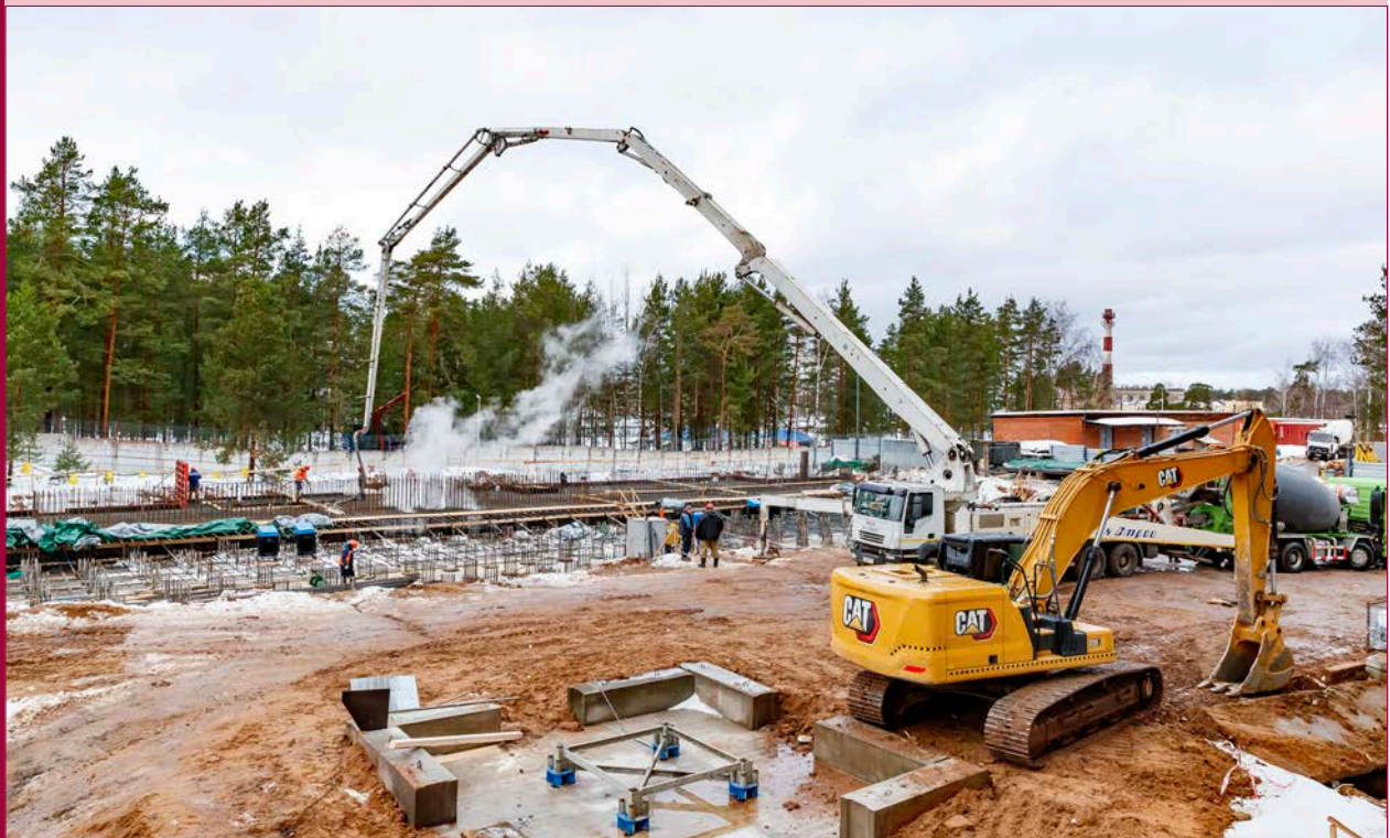
21 December. Pouring the first cubic meters of concrete into the foundation of the U-400R experimental building
