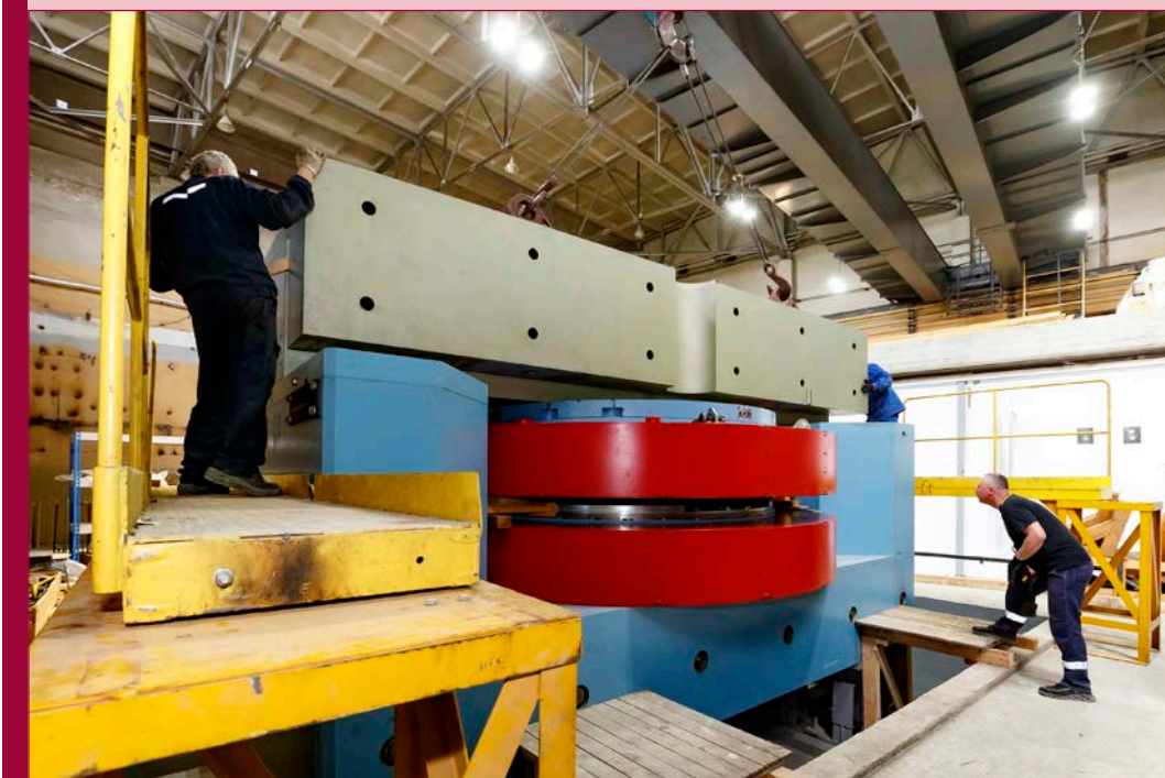
Installation of DC-140
