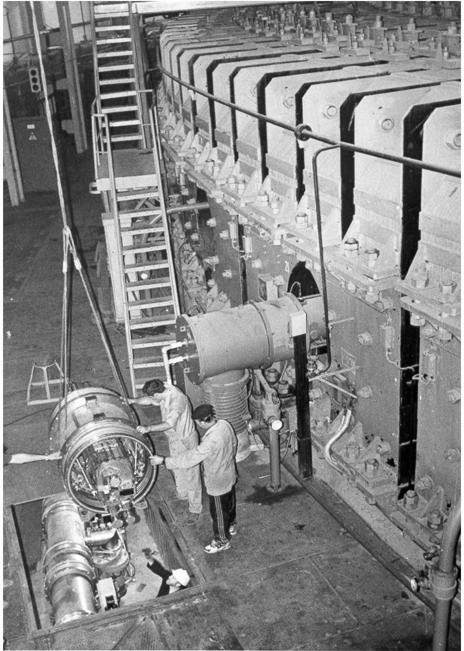
Laboratory of High Energies. Completion of the assembly of the Nuclotron ring's area with elements of the beam slow extraction system
